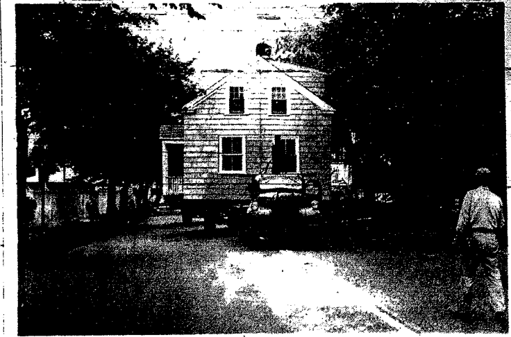
A SECOND HOUSE has been removed from the property owned by Reid Brothers on Elliott street to permit future expansion of the plant. This house is shown above as moved yesterday morning guided it down Elliott street to its new site on Fairview avenue. (Beverly Times Staff Photo)
